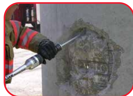
Breaching Concrete
